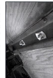
Figure 4-189 Cross Channel Bolts
