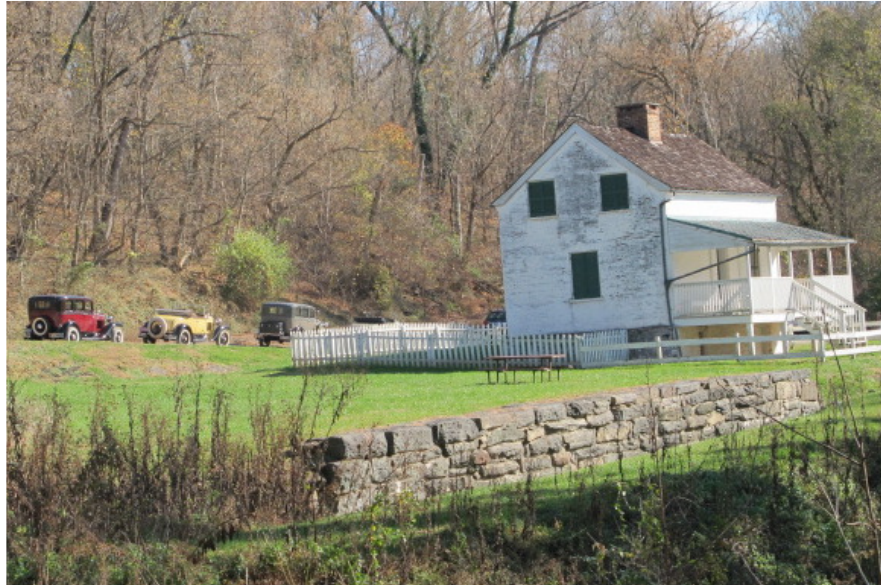
Our A's parked at the entrance to the Catoclin Aqueduct. The house is closed up and not open to the public.
